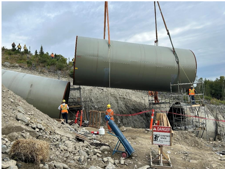
Figure 3: Placing Final Can 28
