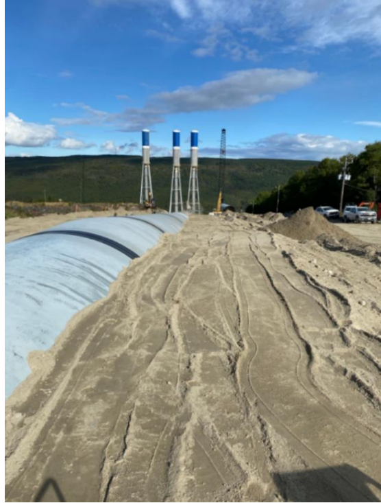
Figure 4: Common Backfill Placement Near Can 14
