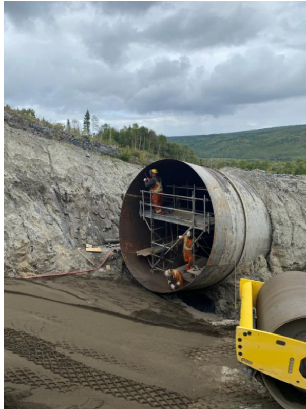
Figure 2: Prepping Existing Penstock at Cut 2 for Can 28 Install
