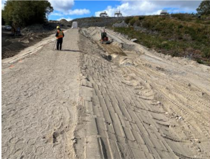
Figure 6: Backfilling and Sloping to Final Grade
