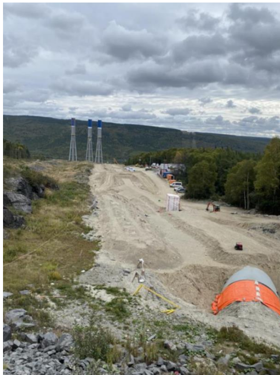
Figure 5: Common Backfill Placement and Sloping
